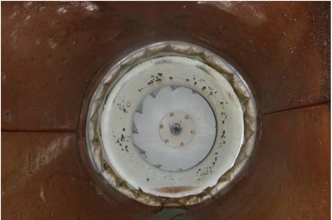
Dried grease buildup in horizontal duct and fan came out very clean.
