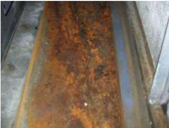
Deteriorated coil pan is quite obvious.
