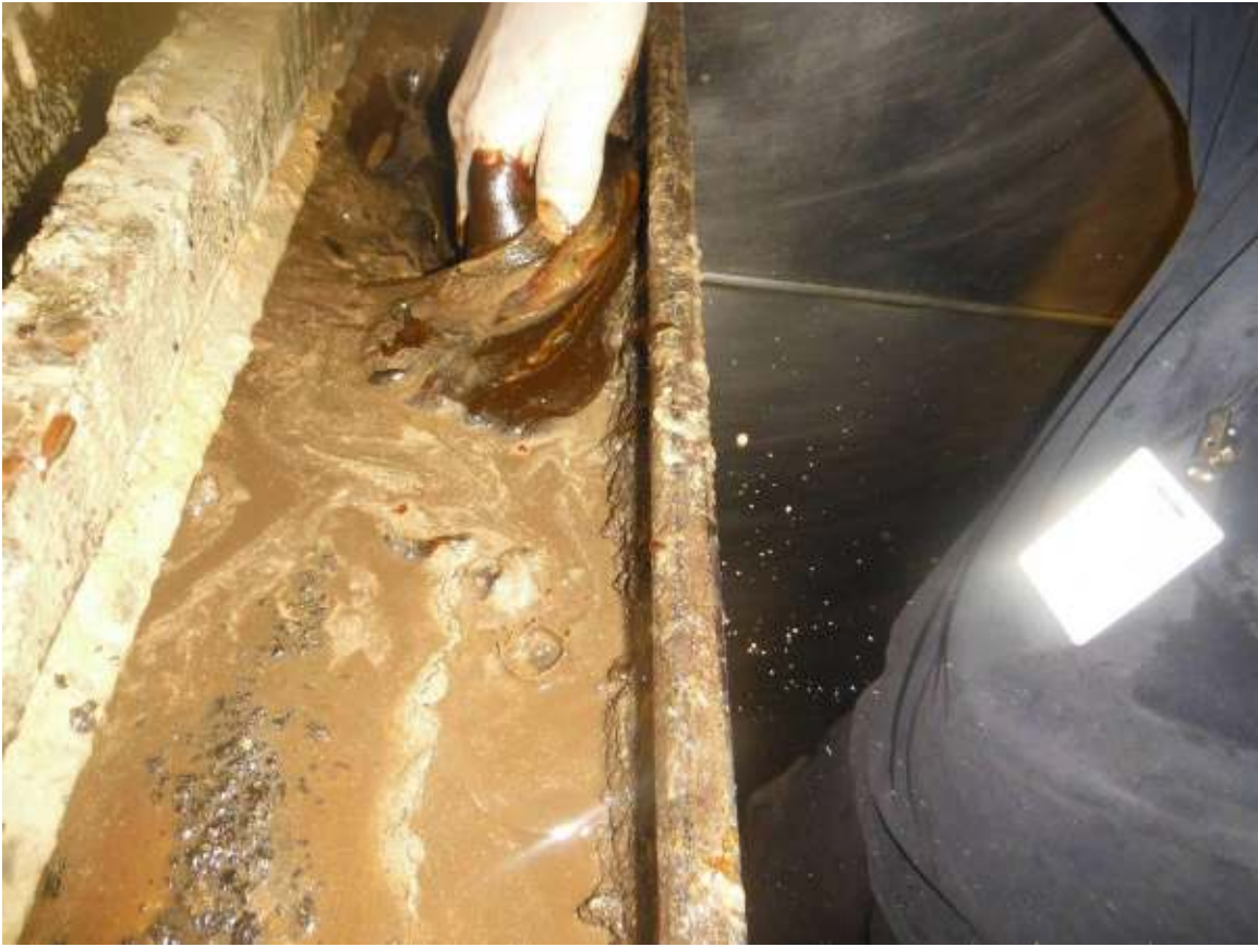
Approximately 100 lbs. of grease was removed during the initial cleaning of the plenums at this facility in downtown Los Angeles!
