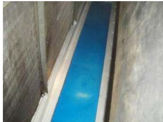
Coil pan after restoration.
