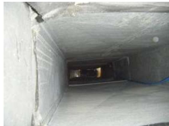
Reverse air duct cleaning tool “flies” down the ductwork, pulling dust and debris back into the negative air.
