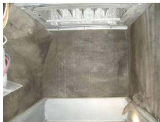
Interior of heating/air conditioning unit after removal of blower, showing deteriorated fiberglass liner.
