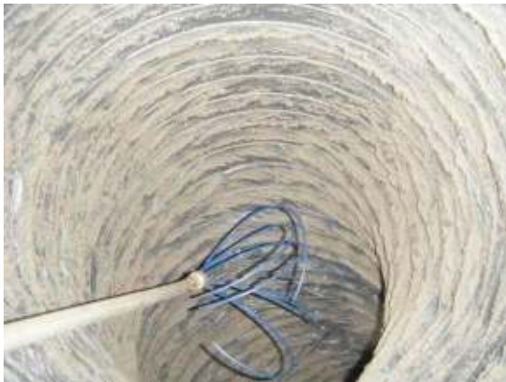
Before use of octopus whip w/negative air pressure
