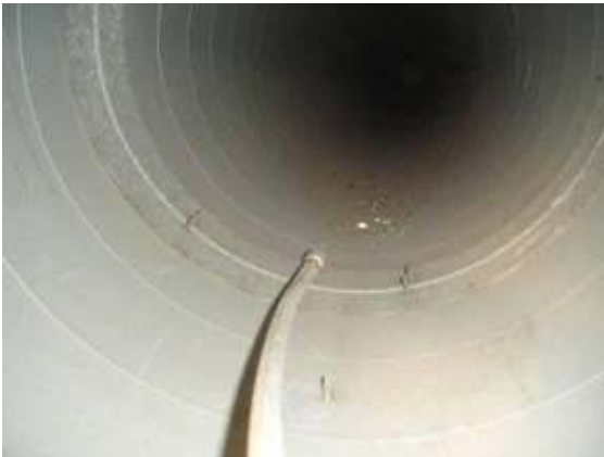
Dust being driven forward into negative air
