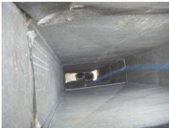
Reverse air duct cleaning tool “flies” down the ductwork, pulling dust and debris back into the negative air.
