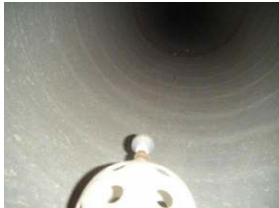
After cleaning with reverse air Scorpion duct ball.
