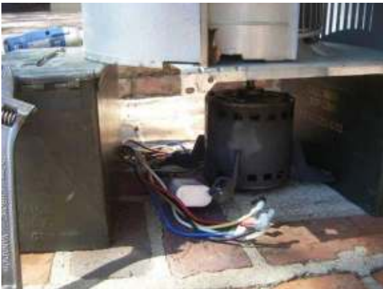
Motors will be disconnected and removed from direct-drive fans, and fans themselves will be taken out and washed with a mild, paint-safe detergent and water, then reinstalled as found.
