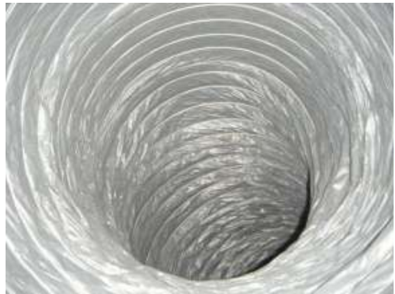
After use of octopus whip w/negative air pressure
