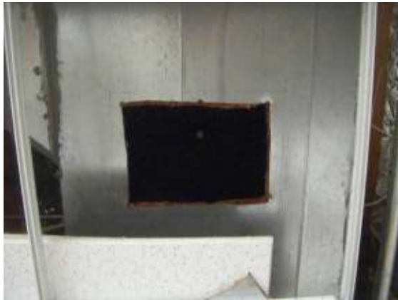
Access holes made in ducts for cleaning purposes are sealed with galvanized sheet metal panels of the same or heavier gauge metal as the duct. Panels are installed with duct sealant and screwed onto the duct at four inch maximum on center all around as required to maintain an airtight seal.
