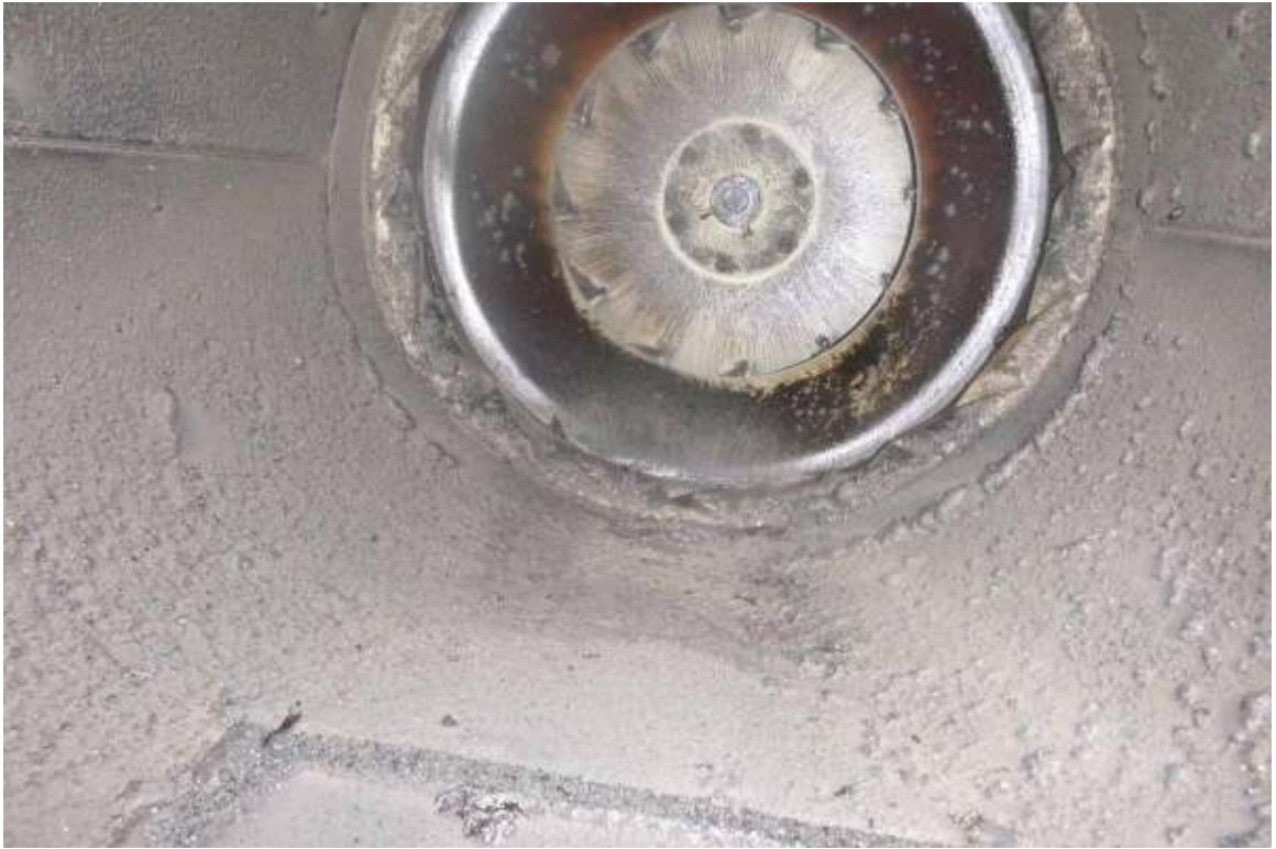
Dried grease buildup in horizontal duct and fan came out very clean.
