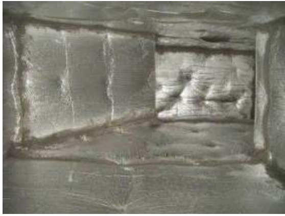
Deteriorated fiberglass insulation can also be overlain with Astrofoil reflective foil insulation.
