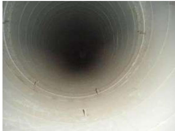
After cleaning with forward air duct cleaning tool
