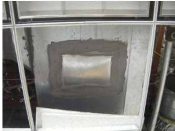
Access holes made in ducts for cleaning purposes are sealed with galvanized sheet metal panels of the same or heavier gauge metal as the duct. Panels are installed with duct sealant and screwed onto the duct at four inch maximum on center all around as required to maintain an airtight seal.
