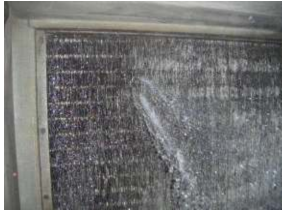
High pressure coil cleaning
