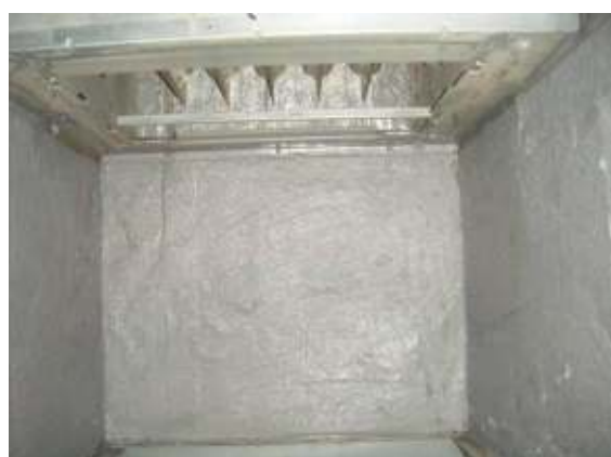
Interior of same heating/air conditioning unit after cleaning and sealing with an anti-microbial coating.
